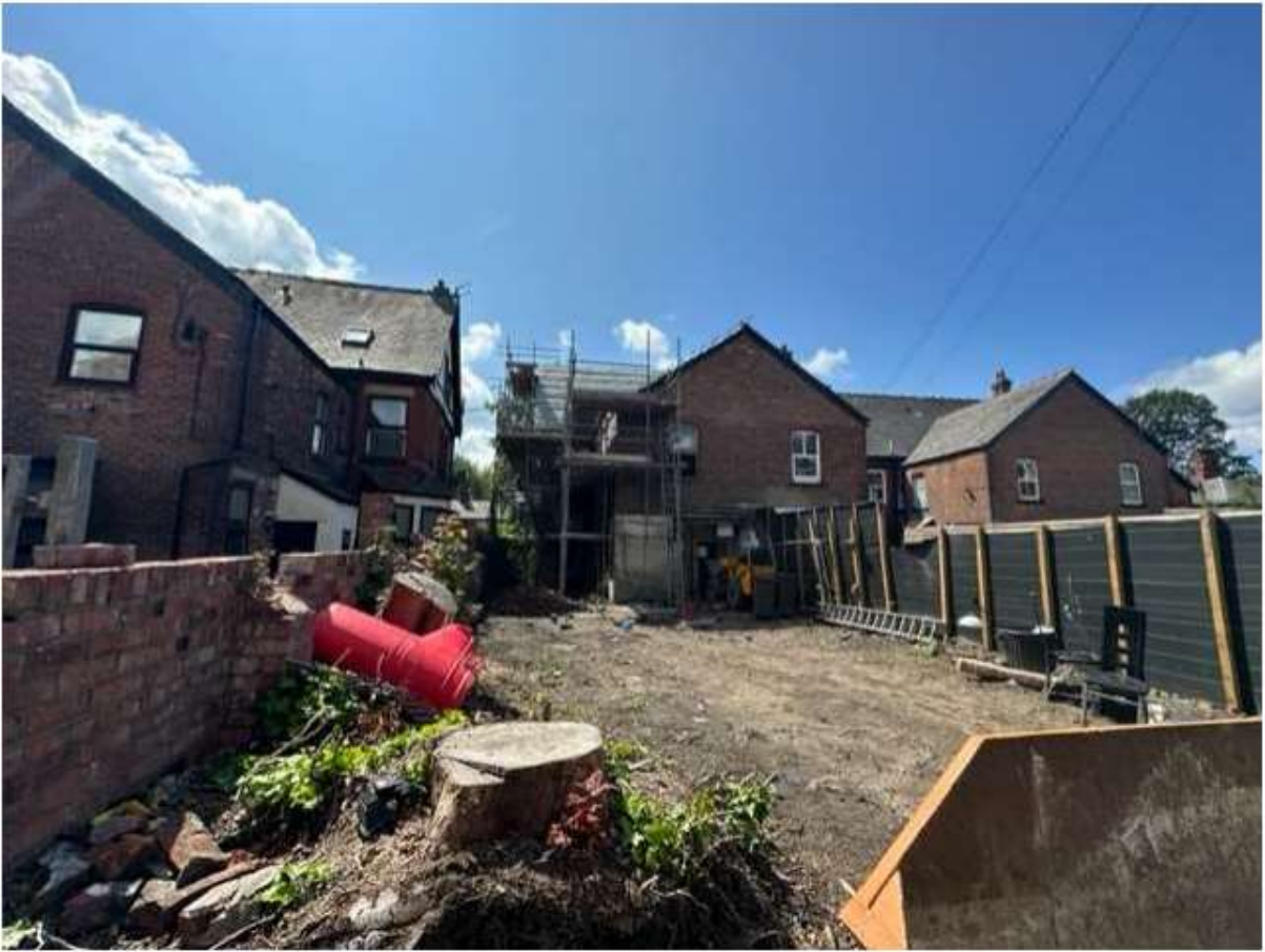
Figure 5 Rear of Property
